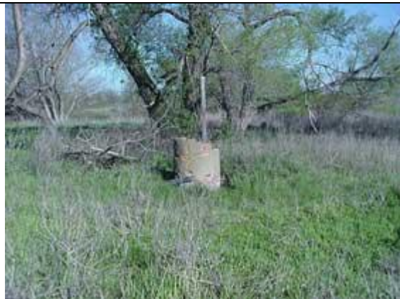
Picture 4. Large Diameter/Hand Dug Abandoned Well
