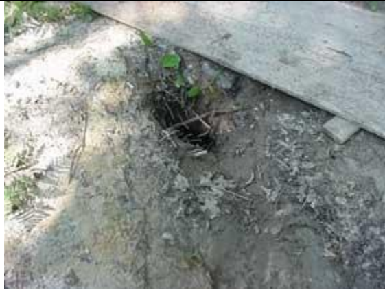
Picture 5. Abandoned well covered with plywood
