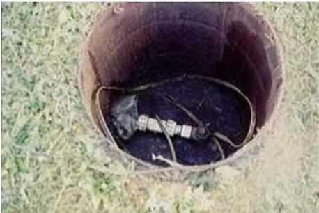
Picture 1. Abandoned well w/casing and pump
