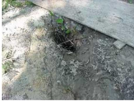
Picture 5. Abandoned well covered with plywood
