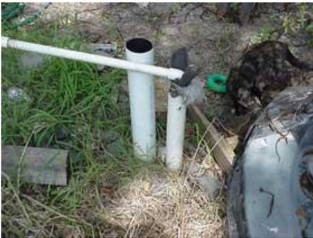
Picture 3. Abandoned well PVC casing.
