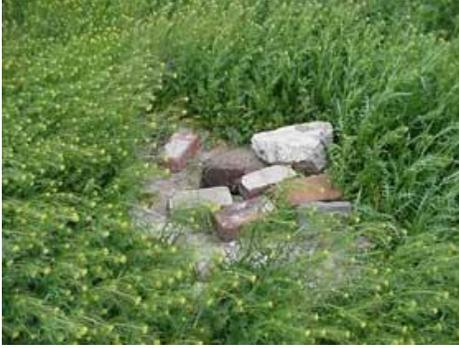
Picture 6. Capped abandoned well with deteriorated casing
